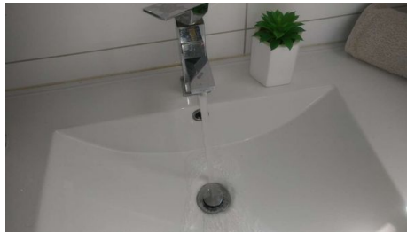
Tap/s Condition: Serviceable condition at the time of inspection
